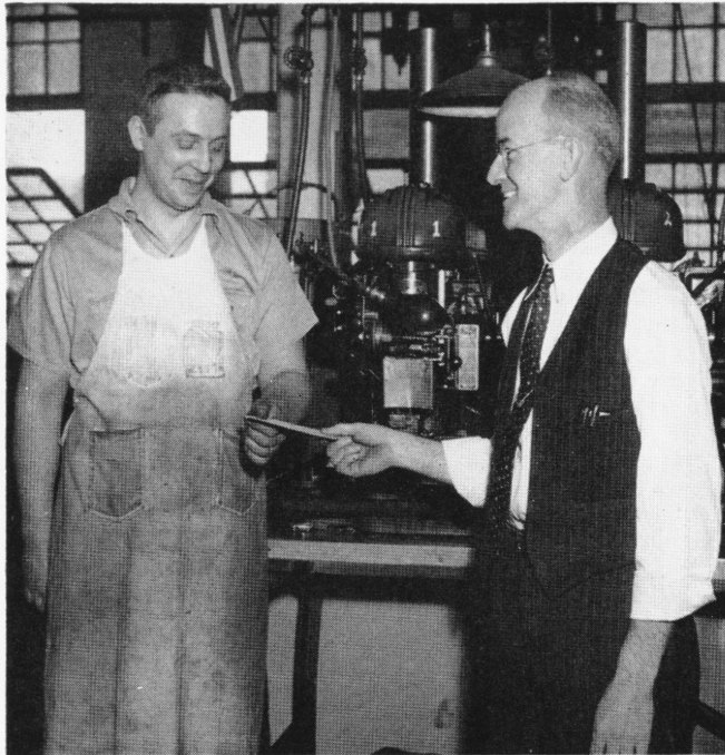
Frank Shanahan, Foreman of the Connector Room, hands Adolph Kudzma, a toolsetter, five dollars in War Stamps for his idea of inserting a small cable through drill press springs to prevent their flying off.
